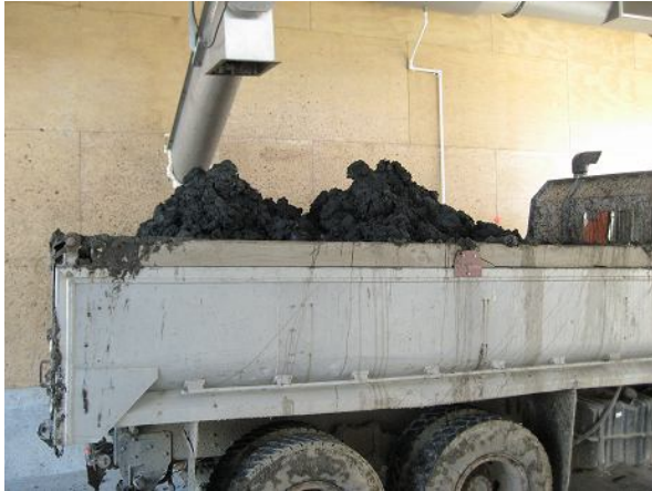
Figure 3: Sludge Auger out-feed to truck
